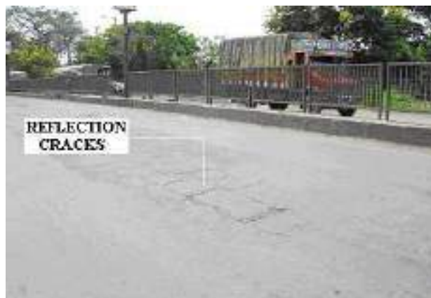
Figure 1. Reflection cracks on overlays with further weakening due to propulsion of secondary cracking
